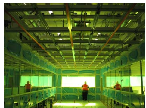
Cleanroom Construction, Photo Bay
